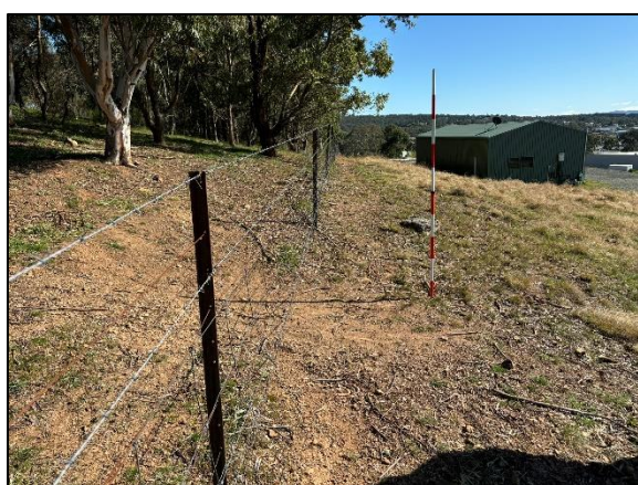
Plate 3. Erosion along upslope fence line (northwest)
