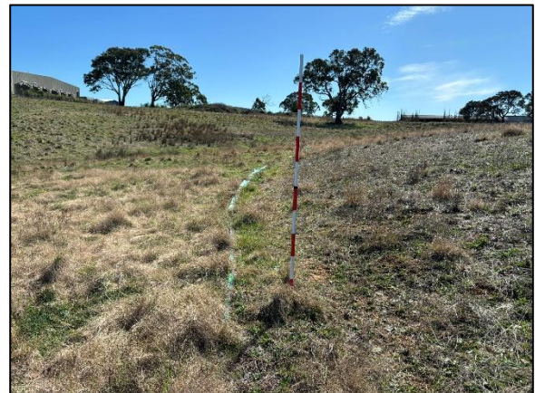
Plate 10. Collapsed erosion control barrier (north)
